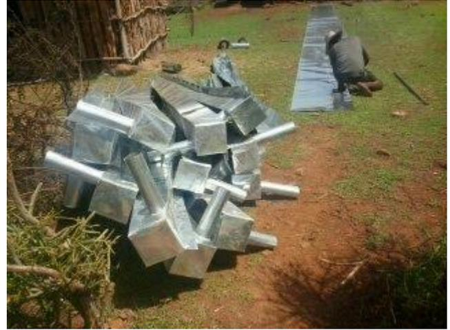
**Picture S3: Perforated pipe for ground water recharge monitoring (left) and collector channel to drain event runoff from plots to runoff tank (right)**
