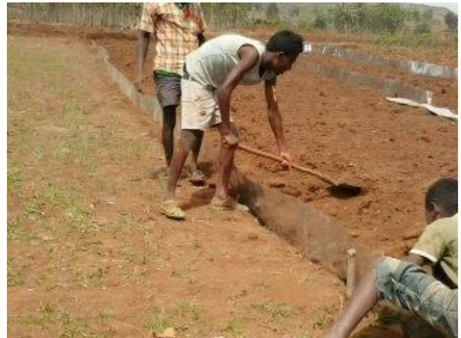
**Picture S8: Trench for sheet metal and plot delineation by sheet metal**
