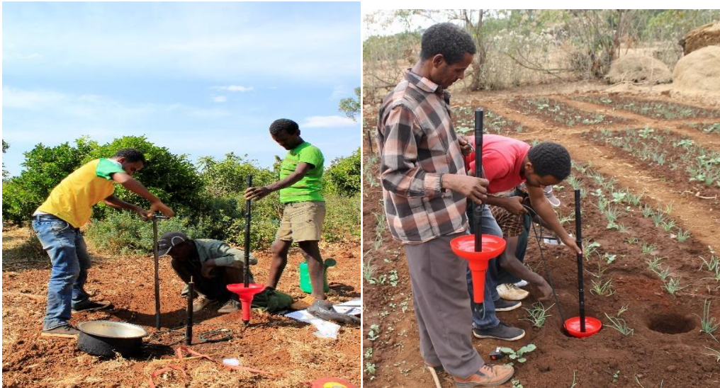
Figure3-4: Installation of Wetting Front Detector at the middle of the plot before starting (left) and changing of the broken WFD (Right).
