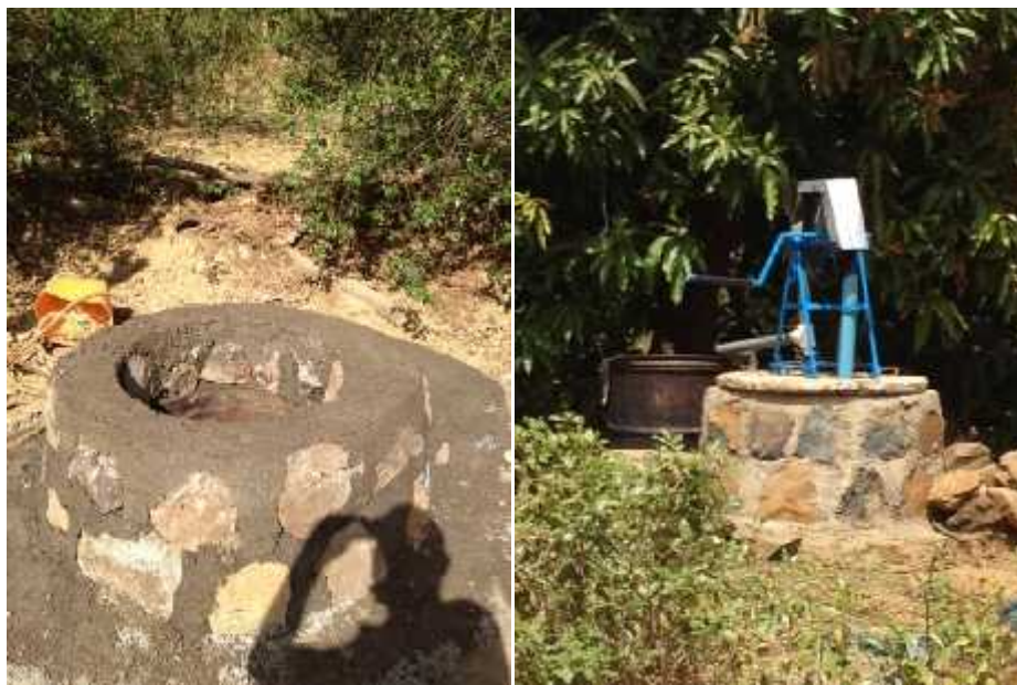
Fig.3.1.1 Shorter rope and washer pump during installation
