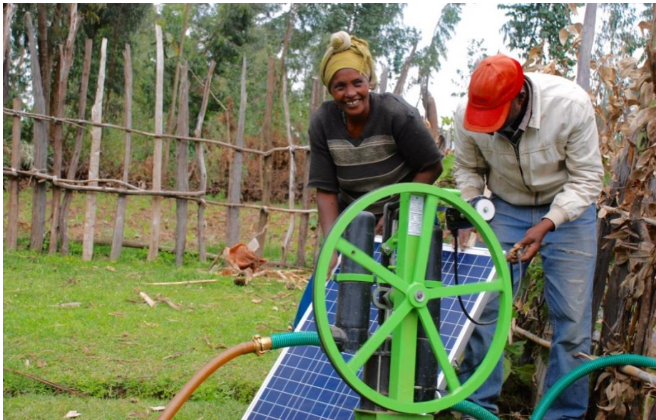
Photo: Installing a solar-based pump in southern Ethiopia. Photo Credit: IWMI
