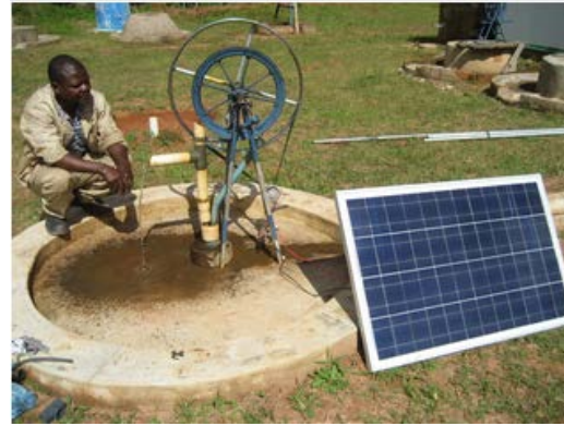
Solar-powered rope-and-washer pump
